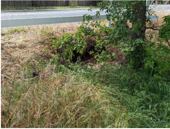
P01 – Culvert looking southwest
